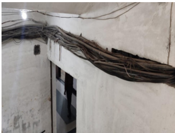
Plate 21. Unmanaged Electrical wiring
