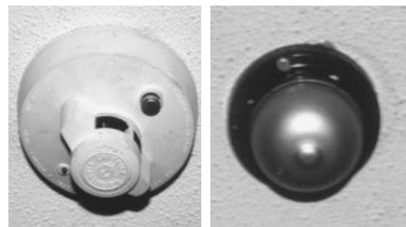
Plate 2. Heat Detector and Smoke Detector
