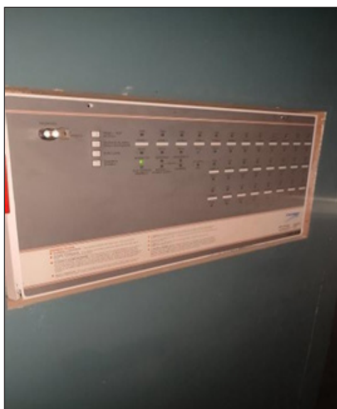
Plate 8. Fire Detecting Board
